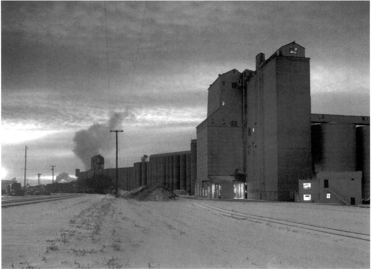
ELECTRIC STEEL ELEVATOR, TWENTY-FIFTH AVENUE SOUTHEAST, MINNEAPOLIS, 1995
